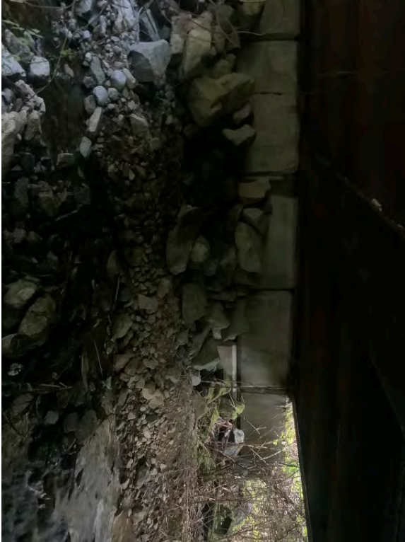
Right Bank Abutment when facing downstream
